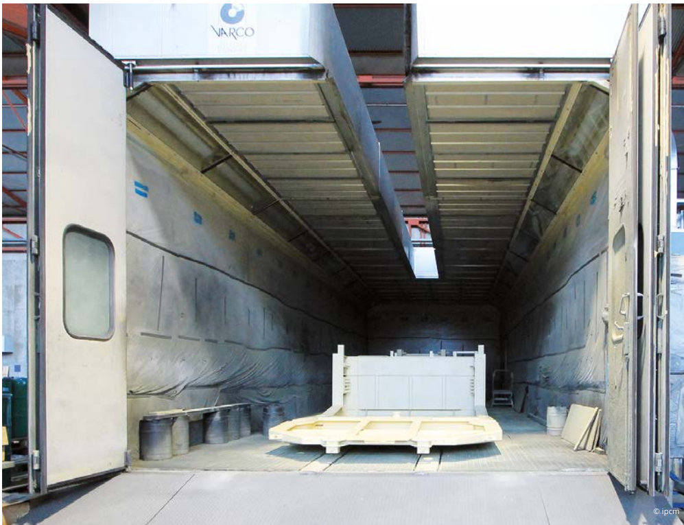
One of the 2 16 x 4.4 m booths integrated with ovens.
