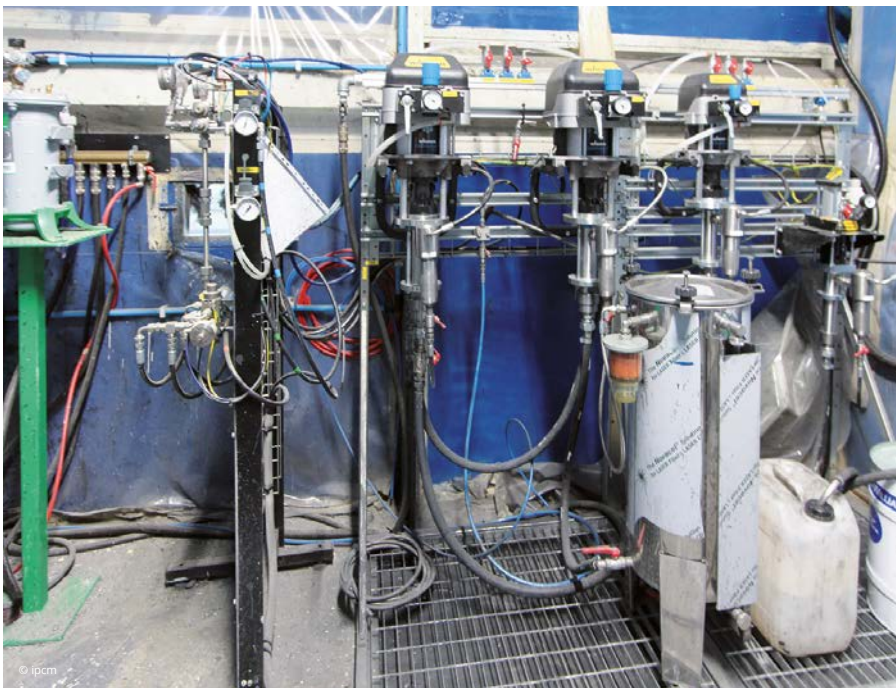
The paint management unit with Wagner mixing pumps.
