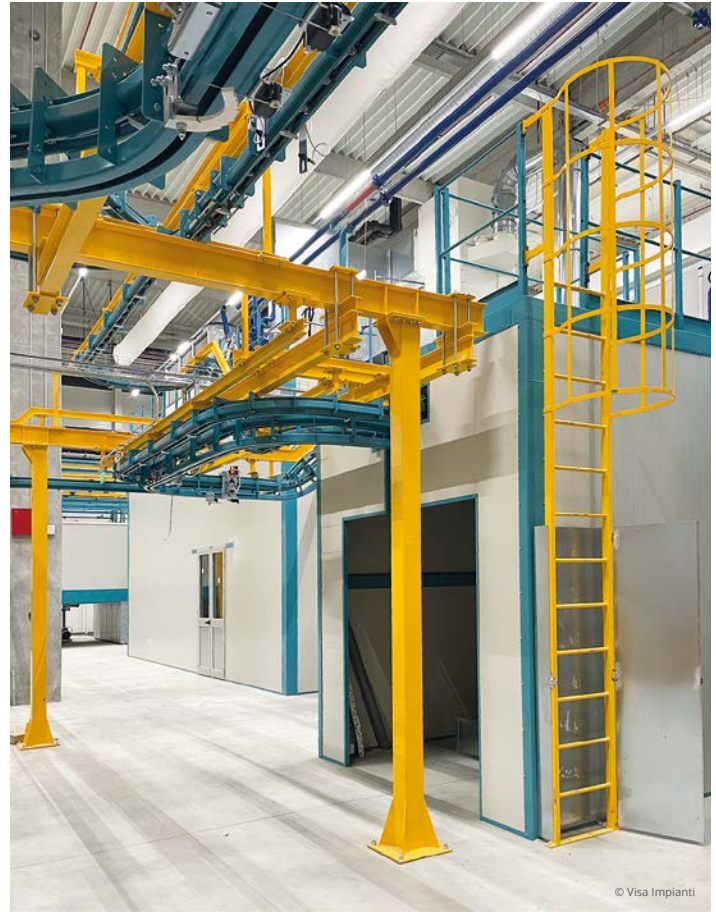
A detail of the coating system provided by VISA Impianti.
