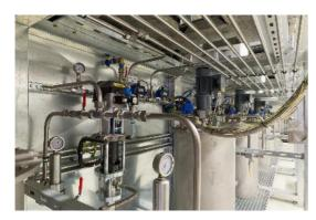
Seven Puma 8-300 pumps from WAGNER transport the components at low pressure from the paint supply room to the painting booths. To be able to bridge the large distances, Thüma has installed an innovative loop line with a switchover between the flow and return pipe.
