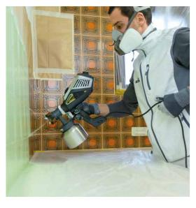
Another question for the professional painter: how can I quickly paint old tiles in one application? Since Pierre sprays in a cross-coat pattern, i.e. first from top to bottom and then from left to right, he gets more paint on the tiles. This means he applies a thicker layer of paint and can cover the tiles in a single application. To do this, he changes the spray jet, so he always has the right paint jet for his working direction.
