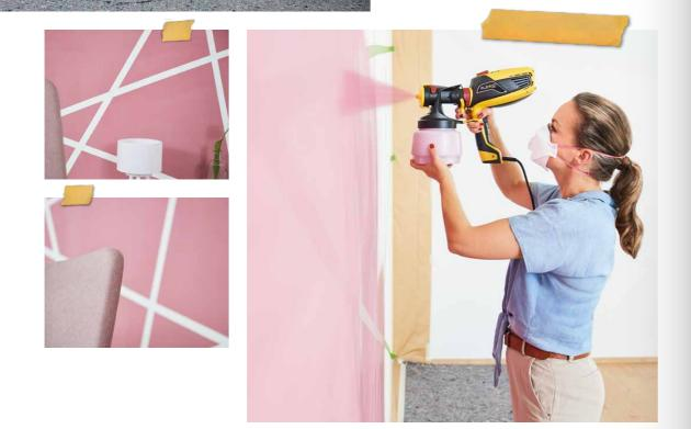
If you've decided on painting a relatively large wall, ask a second person to help with the masking work. This saves time and is also twice as much fun! Sticklers for precision can mark out the pattern in advance using a pencil and a laser spirit level. This projects a straight laser line at the desired angle on the wall and then it's simply a case of aligning the masking tape.
