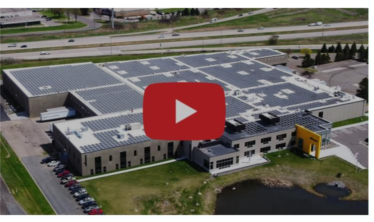
The WAGNER Group subsidiary in the USA, Wagner Spray Tech Corp., has installed the largest solar system currently available in the US state of Minnesota on its new roof. 3,700 individual panels produce 1,643,000 kWh per year. This amount would cover the average annual power consumption of 410 German four-person households. Efficiency and sustainability are important to us not only in our products but also in our companies.
